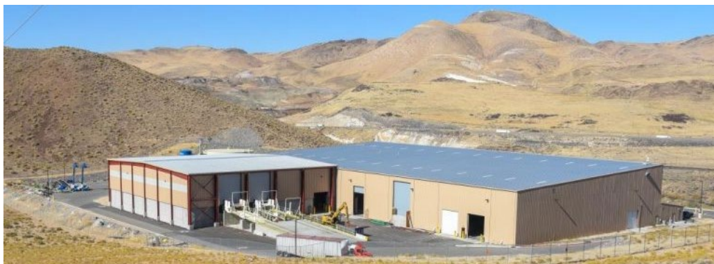
Fulcrum bioFuels plant located in Nevada, USA Strategically located adjacent to waste landfill
